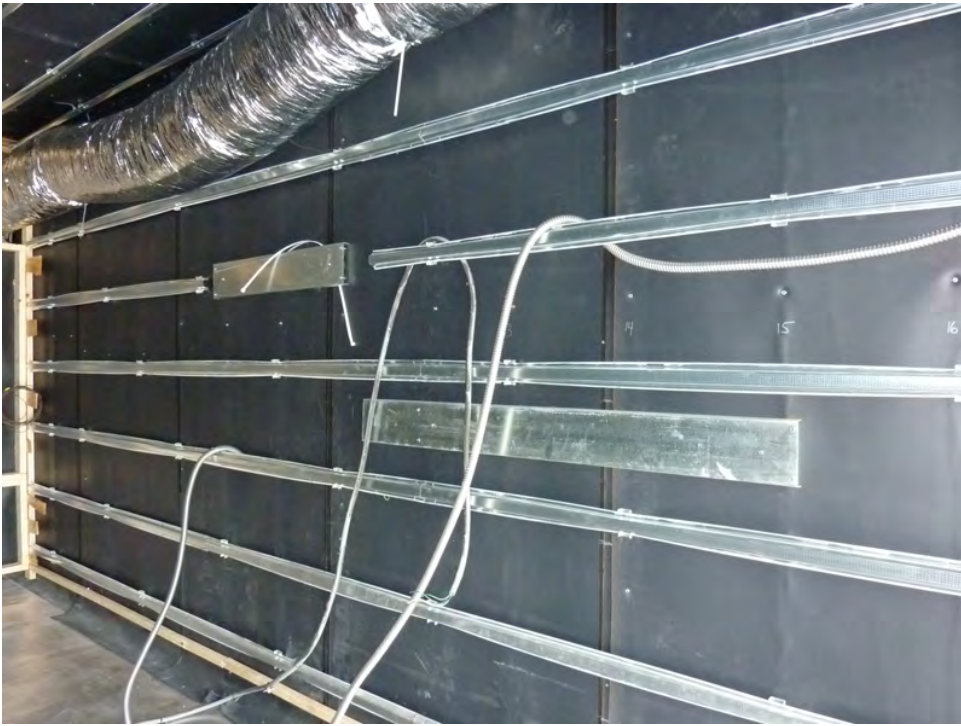
Interior Wall Isolation - RSIC-1 Iso Clip with High hat channel
