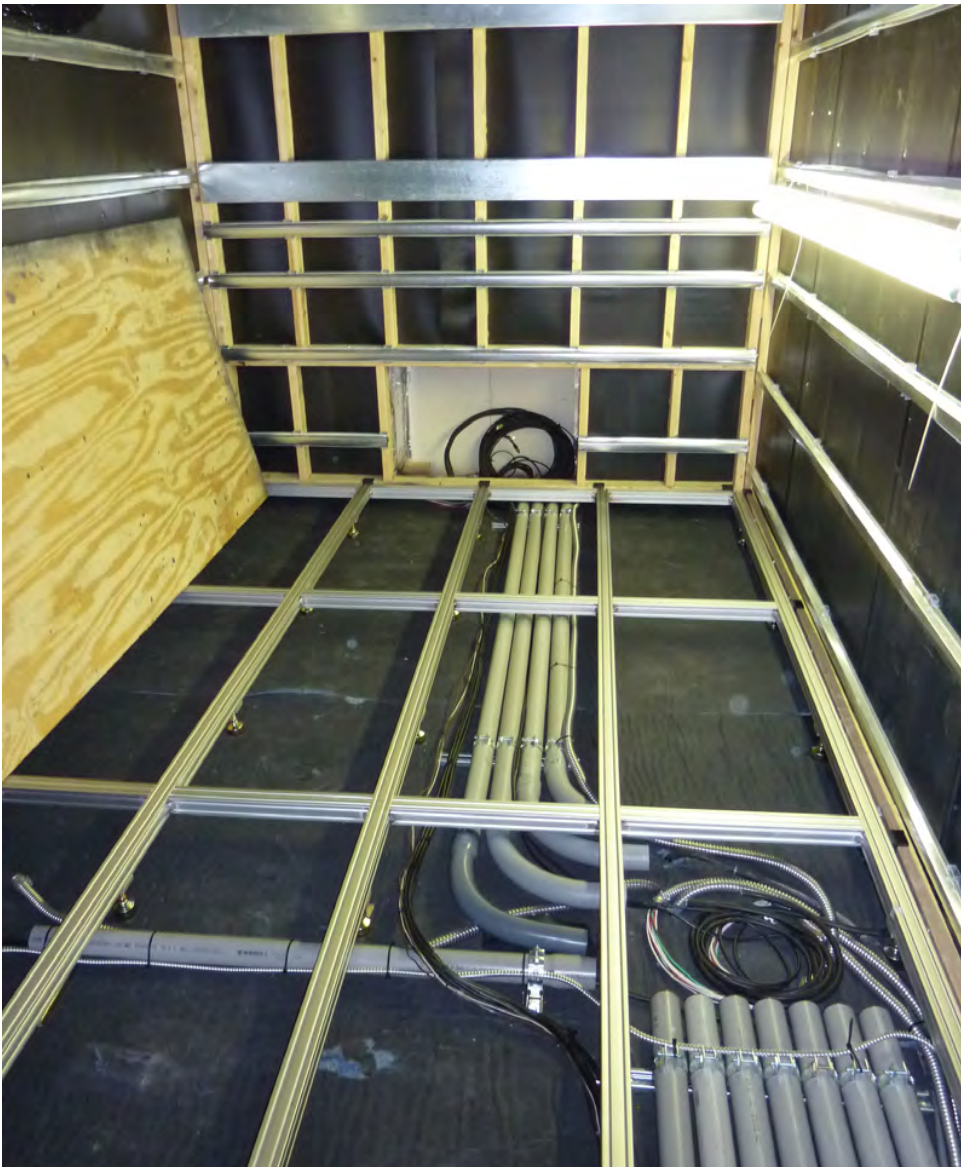
Floor Isolation - Suspended aluminum structure with Quiet Liner Acoustic Sound Sealant on all edges and corners.
